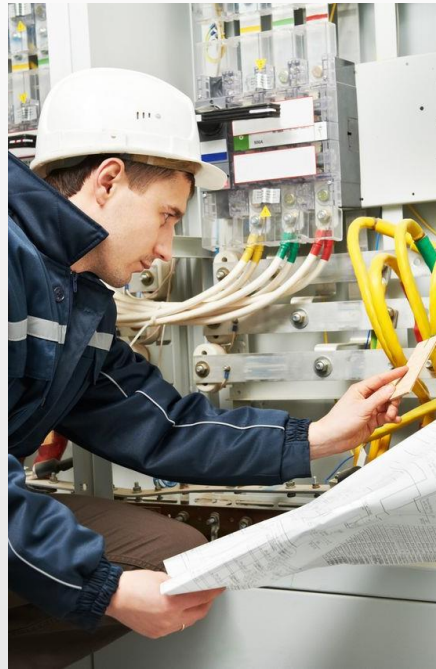
Service and Revamping
